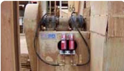
Lubricator: perma Star Vario Bracket: MB02 with BC30 Install Kit: K230 Ref #: FAN02
