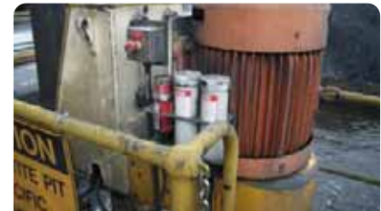
Equipment: Warman sump pump perma Star Vario MB03-C with BC30 Lubricator: perma Star Vario MB03-C with BC30 Bracket: K330C Install Kit: K330C Ref #: PUMP06
