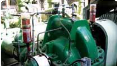
Equipment: Pump perma Star Vario Direct Lubricator: perma Star Vario Direct Bracket: Direct Ref #: PUMP07
