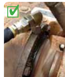
perma Star Vario providing a constant grease purge to the labyrinth seal of a Warman pump, thereby protecting against water ingress.
