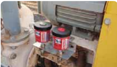
Equipment: Warman pump perma Futura MB02 with BC30 Lubricator: perma Futura MB02 with BC30 Bracket: K230G Install Kit: K230G Ref #: PUMP04
