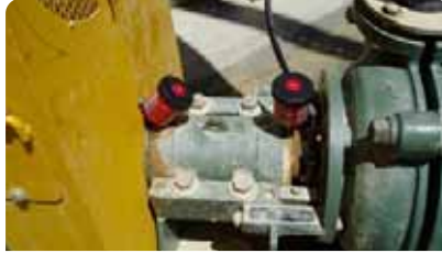
Equipment: Warman pump perma Futura Direct Lubricator: perma Futura Direct Bracket: Direct Ref #: PUMP02
