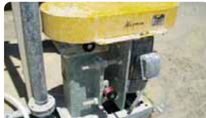
Equipment: Warman sump pump perma Futura Direct Lubricator: perma Futura Direct Bracket: Direct Ref #: PUMP05
