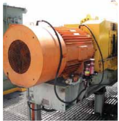
Lubricator: perma Star Vario Bracket: MB02 with BC30 Install Kit: K230 Ref #: MOTOR03
