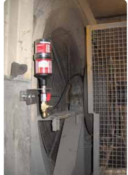
Lubricator: perma Star Vario Bracket: MB01 with BC30 Install Kit: K130 Ref #: FAN04
